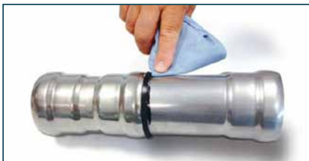
Figure 8 - Cleaning of the grease residual
