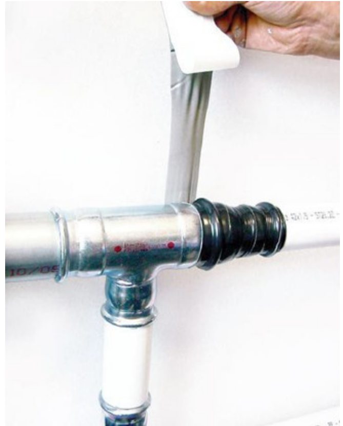
Figure 34 - Protection of the connectors with butanol adhesive tape
