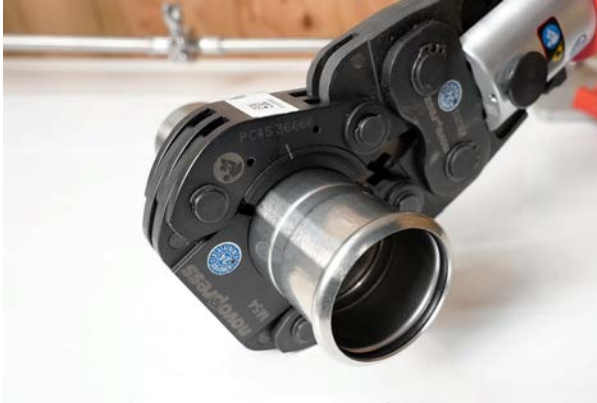
Figure 28 - Making the press connection
