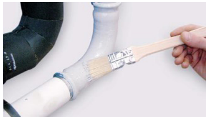
Figure 33 - Varnishing of the connections and tube with primer.
