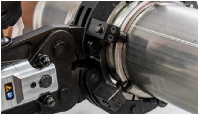
Figure 31 - Press assembly phase 2
