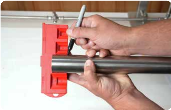
Figure 25 - Marking the insertion depth
